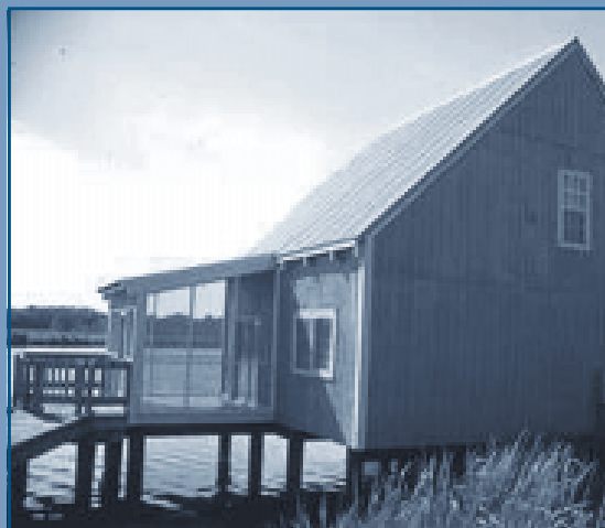
Cabin at Bayou Segnette State Park
